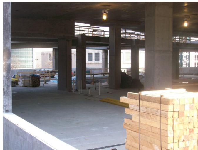
Figure II.II – Lobby Level during Tower Erection
