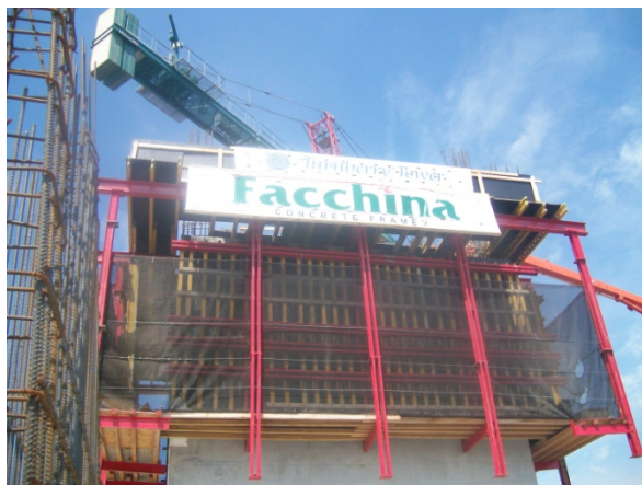
Figure III.II – ACS Formwork for Core
